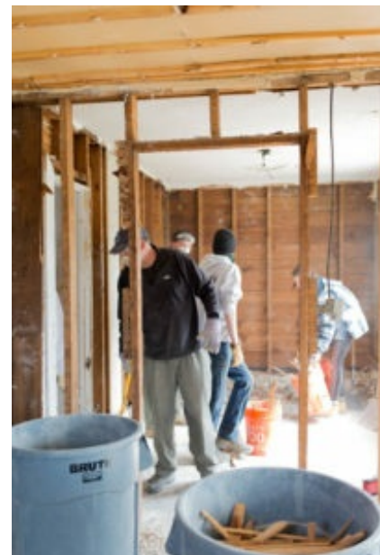
Volunteers working on a house adjacent to the church
